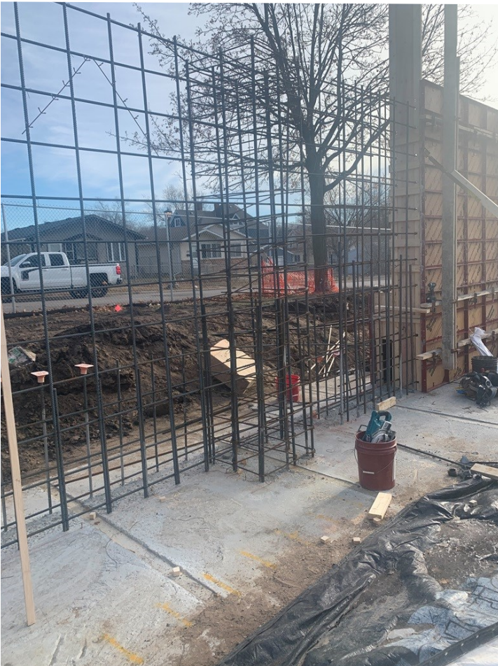
Top row: Framing up the wall panels; Second row: Rebar for wall panel; wall poured (December 2023)
